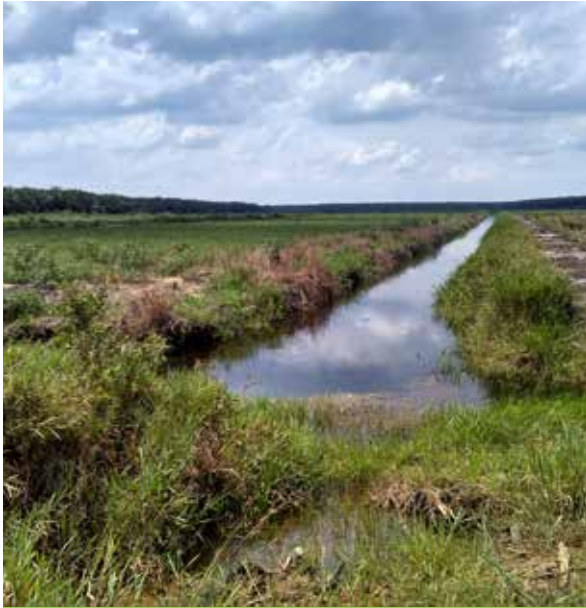
Canals dug to drain peatland before planting palm oil trees are blamed for drying out the peatland
