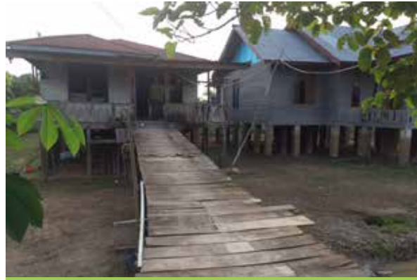
People build raised houses in Jambi to avoid regular flooding, noted as a greater problem than haze
