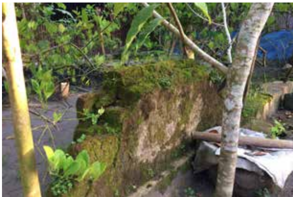
A wall from this family's previous home which was destroyed during the earthquake. The father said they've kept it as a 'memory'.
