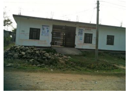
VDC building in Morang closed due to recent conversion to Municipality
