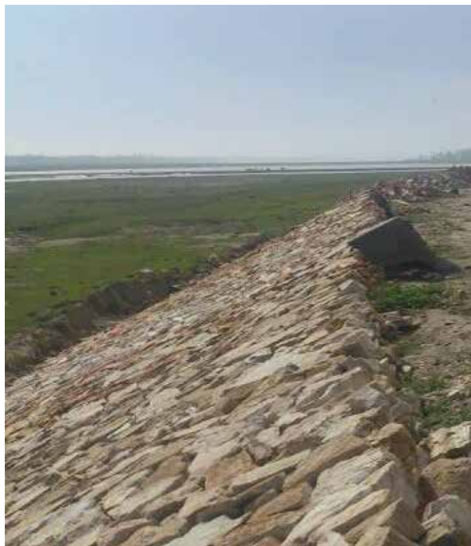
Retention wall being built to mitigate future floods in Nowshera river.
