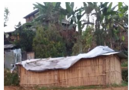
Temporary shelter constructed 3 days after the first earthquake in central Dhading
