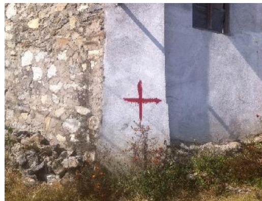
A red cross put on a house in the Kathmandu Valley by a technical team in to identify it as 'fully damaged'
