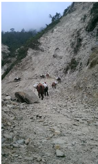
Trail in upper Gorkha damaged from landslides
