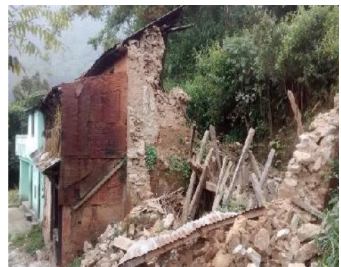
A damaged house in Kathmandu Valley
